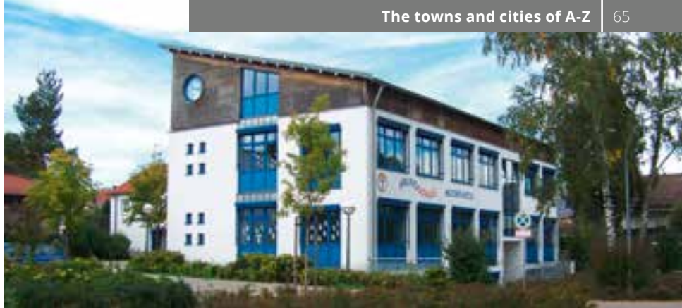
Primary School Moorenweis. Photo: Municipality of Moorenweis
